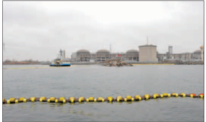
OPG employees work by boat to install a fish net at Pickering Nuclear in April 2011.
