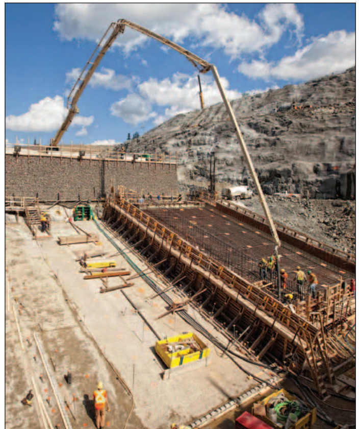
Rebar instalment for the intake structure at Smoky Falls GS.
